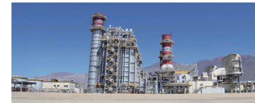
Kelar gas-fired combined-cycle power plant
